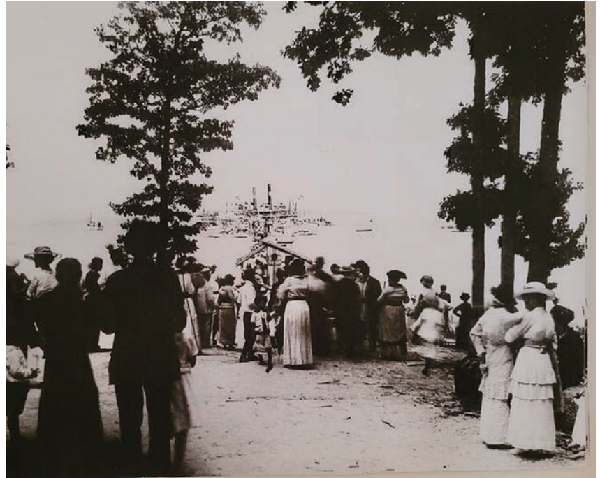
Wharton Grove Wharf on the Corrotoman River was about a quarter mile long and very busy during camp meeting days. The wharf was demolished in a 1933 storm and replaced by a 300-foot dock. Written on the back of the photo is "This is of a camp meeting near here. This is a great place for motor boats and pretty girls. A.D.D." Photo courtesy Steamboat Era Museum
