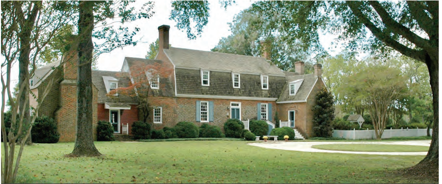
Verville, approaching from the north, the center portion of the house is the original 1725 construction. In the early 1800s, Judge Ellyson Currie expanded the home's footprint by adding an east wing library on the right, which is hidden behind the small north wing office added during the same period. He also added a west wing pantry, which is now a kitchen, on the left. The most recent additions were made by the Duntons—a porch off of the east wing, also hidden by the office, and extending the west wing to include an informal dining room and bedrooms. The house was listed on the Virginia Landmarks Register in 1986 and the National Register of Historic Places in 1987.
