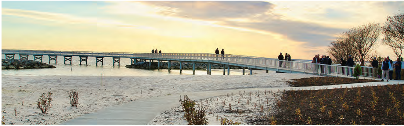
A restored and revitalized Westland Beach in Lancaster County officially opened in November 2025. The 15-month, $4.8 million project restored the beach using 16,000 cubic yards of beach sand recovered from dredging the nearby marina channel. A series of jetties were constructed to protect the existing beach and allow more sand to naturally build. About $2 million of the project came from state and federal grants related to flood preparedness and small watersheds. Other amenities include—a 450-foot long pier on the Rappahannock River with fish cleaning stations; feet washing stations at each end of the public beach, public restrooms, and a 50-space parking lot. All features are compliant with the Americans with Disabilities Act. Master plans were designed by GuernseyTingle Architecture and LPDA Landscape Architecture. Engineering was provided by Bay Shore Design and Bay Design Group. The beach restoration and pier installation was provided by Docks of the Bay. The parking lot, restrooms and boardwalk were constructed by Norman Company. Photo by Jackie Nunnery
