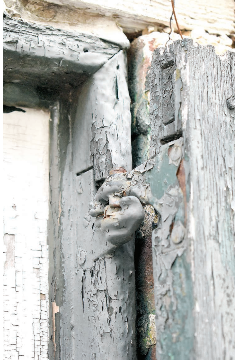
Although covered in layers of paint, this was the only original shutter hinge on the windows. The rest had been replaced over time.
