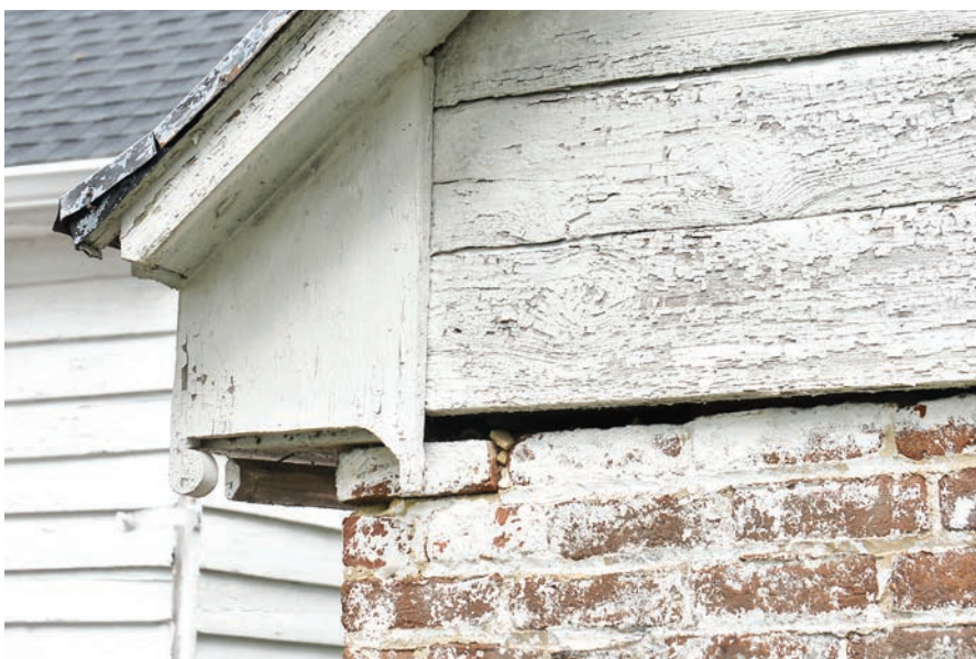
The only undamaged and original outside ornamental corner molding on the dairy is shown in this photo. The other three corners of the building show that time and elements have damaged the wood molding.
