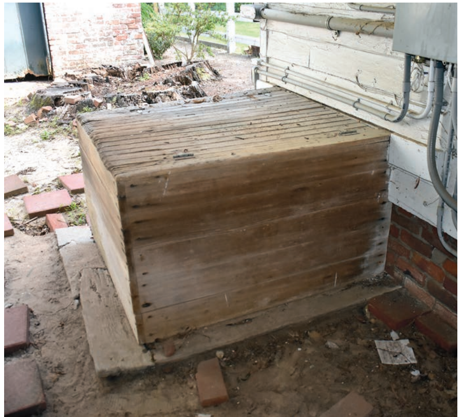
This milk and butter box at Walboro leads to a dry well about six feet deep. A dumbwaiter was used to lower and raise food items in and out of the dry well. The box and dry well is a classic 19th century refrigerator.
