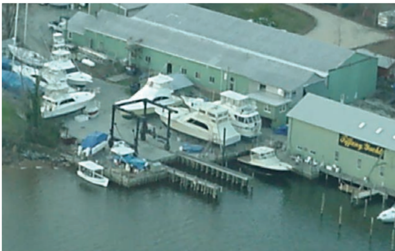
Prior to the devastating fire in 2010, most maintenance and production was conducted in this large building. Photo courtesy of Tiffany Yachts
