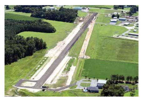
A major project was recently completed at Hummel Airport in Topping where the runway was lengthened 1,000 feet and realigned so planes do not need to fly over homes. New asphalt can be seen next to the old runway, which has been removed. A public-private partnership funded the project at no cost to Middlesex County, which owns the airport. Photo contributed by Nancy and Richard Lewis
