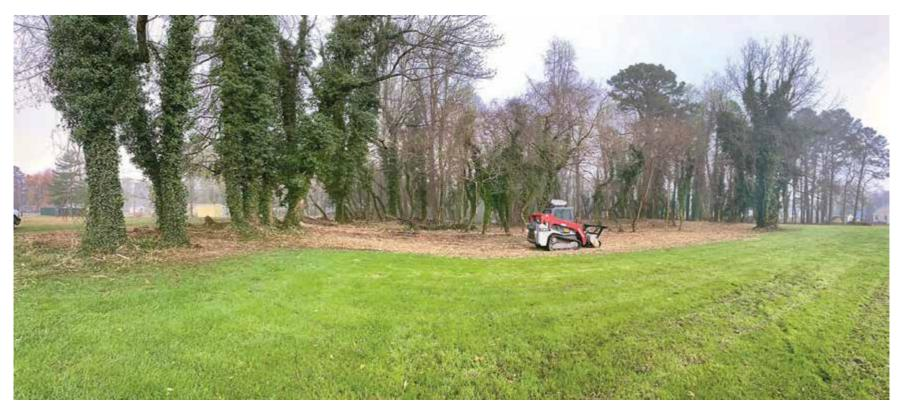
When the business of clearing an area is complete the Takeuchi Mulcher leaves the ground covered in a layer of mulch. There is also no ground disturbance which means no permits are required to do the work. This photo was shot on Rappahannock Avenue in Urbanna on land owned by the Urbanna Oyster Festival Foundation. Photo by Brian Fletcher
